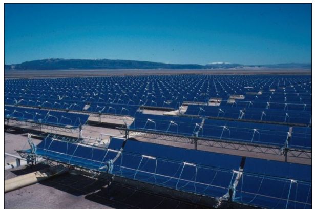
Parabolic trough collector field for the solar thermal power plant at Kramer Junction, California
